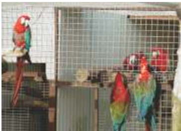
Figure 11. Typical construction of the aviaries involved in the study. The wood and galvanised wire construction made disinfectant application difficult.
